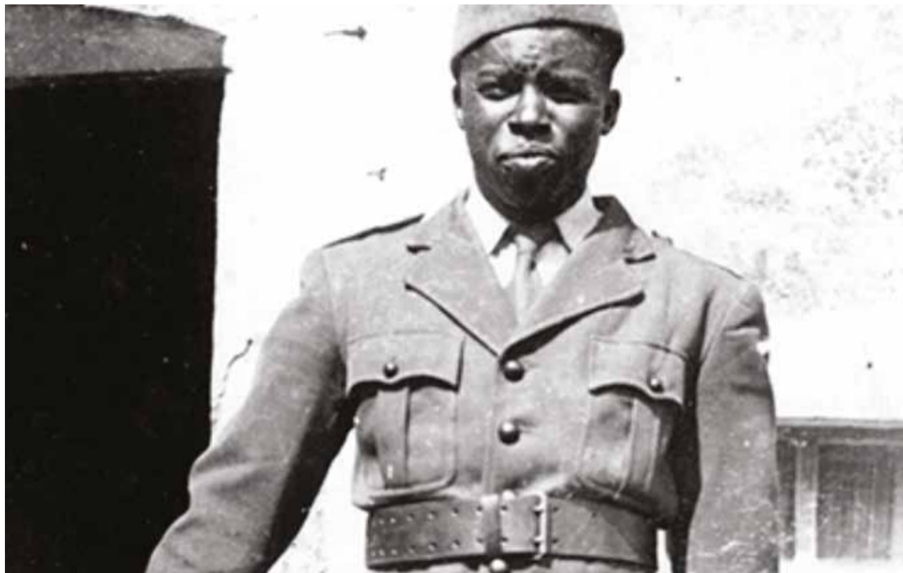
Addi Bâ in Tollaincourt, 1943
